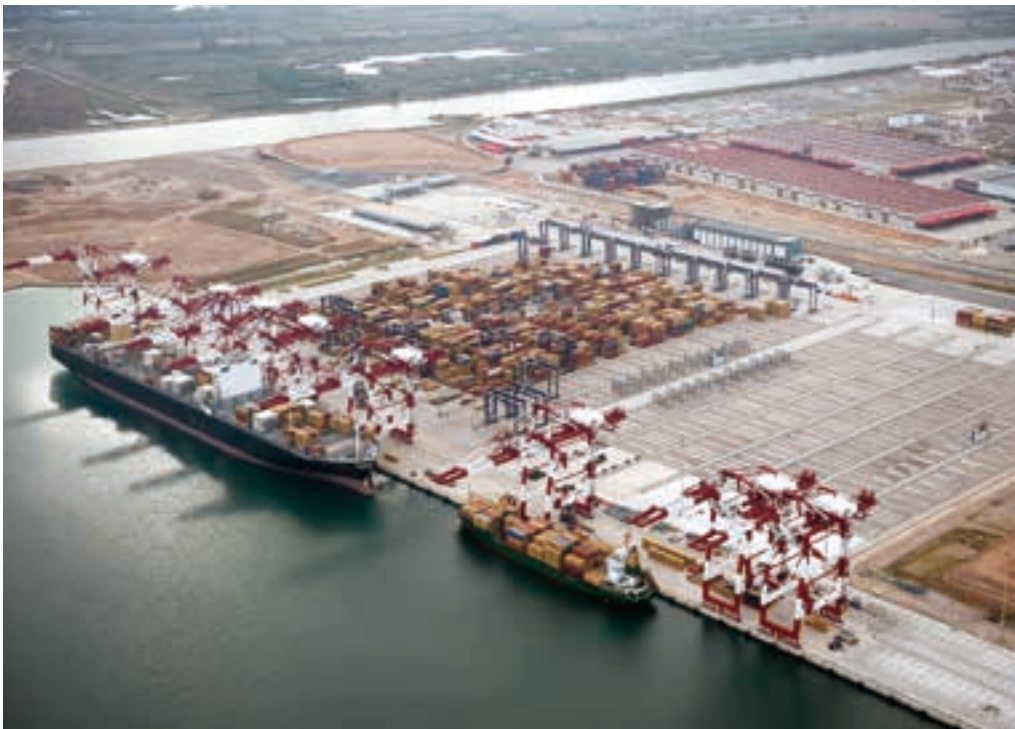
The semi-automated Barcelona Europe South Terminal is the most technologically advanced port facility in Southern Europe.
