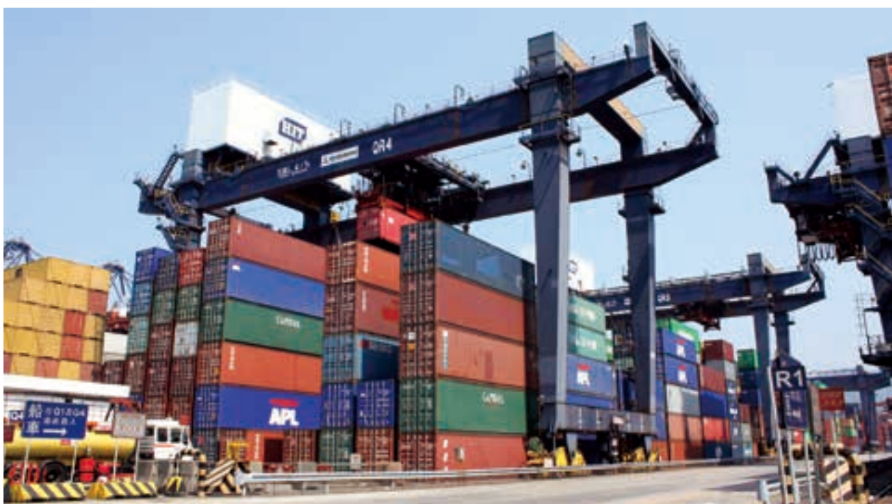
HIT is in the process of installing remote control stations for its fleet of 24 Rail Mounted Gantry Cranes.
