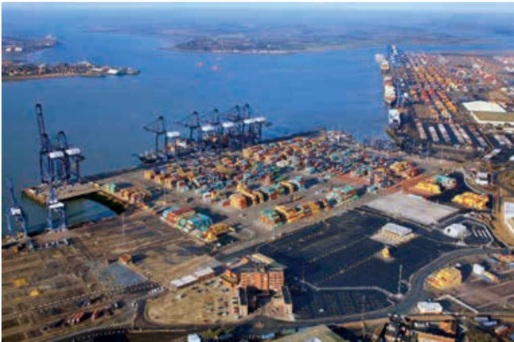
The first phase of Port of Felixstowe's Berths 8 and 9 provides the deepest draft available at any UK container port.
