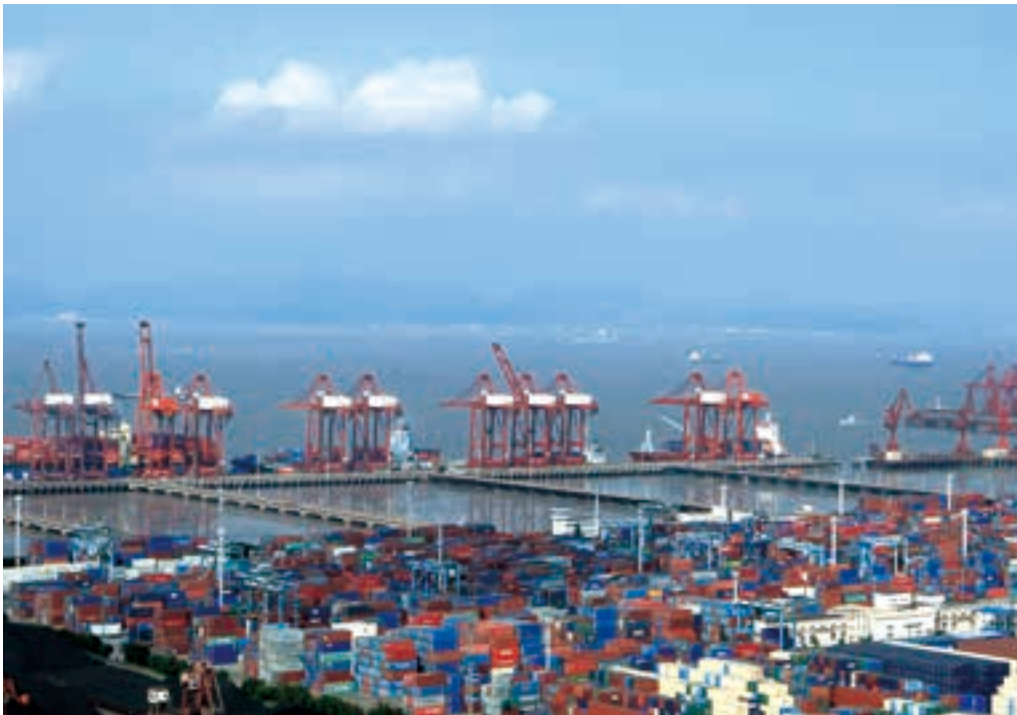
Ningbo Beilun International Container Terminals is a natural deep-water port with a depth alongside of 18.2 metres.
