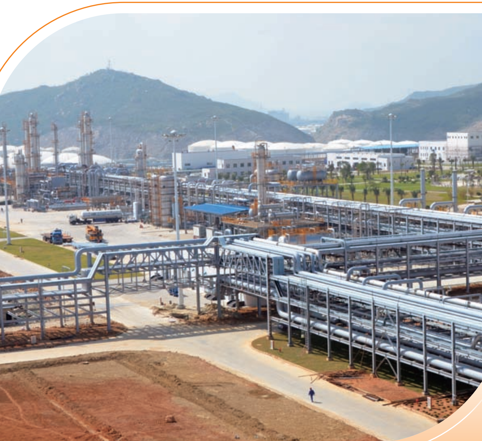
The Gaolan Gas Terminal, in the Mainland, processes the gas and gas-liquids from Liwan 3-1 and Liuhua 34-2 fields.
